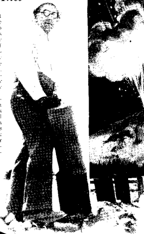
Fred G. Hitt, engineer in charge, placing bombs used in the man-made eruption
