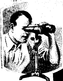
Field glasses with lapel microphone attached to lenses so announcer can talk and watch game
