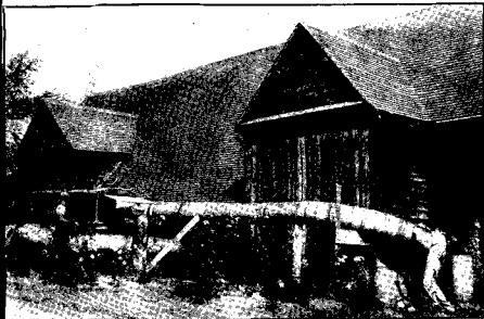
Barn near Beaconsfield, England, that supplied the timbers for the famous ship, Mayflower , is being saved from ravages of death watch beetles with hot air pumped into it through big pipes.
