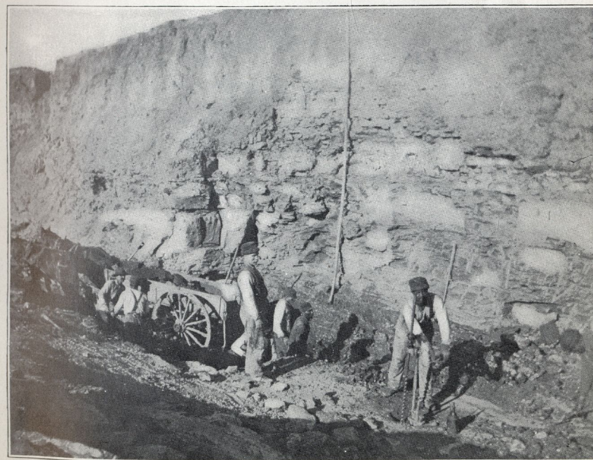
STRIPPING COAL AT LEHIGH, IND. T.
