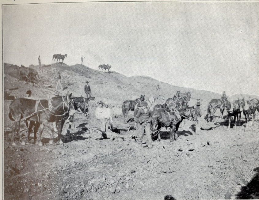
STRIPPING COAL AT LEHIGH, IND. T.
