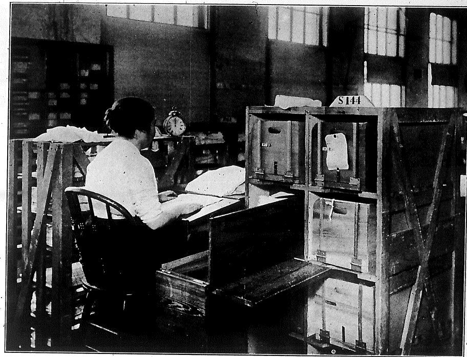
Fig. 14. Standard Work-place, Trucks and Containers for Folding Handkerchiefs.
