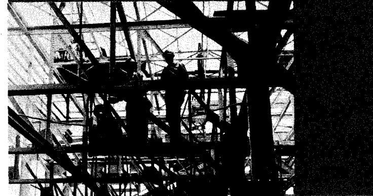
NUMBER THREE. Structural steelmen work on the cooling tower of the Inland's third continuous galvanizing line at Indiana Harbor. This new line, rapidly nearing completion, will substantially increase Inland's production of TI-CO galvanized sheets.
