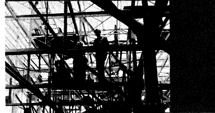
NUMBER THREE. Structural steelmen work on the cooling tower of the Inland's third continuous galvanizing line at Indiana Harbor. This new line, rapidly nearing completion, will substantially increase Inland's production of TI-CO galvanized sheets.
