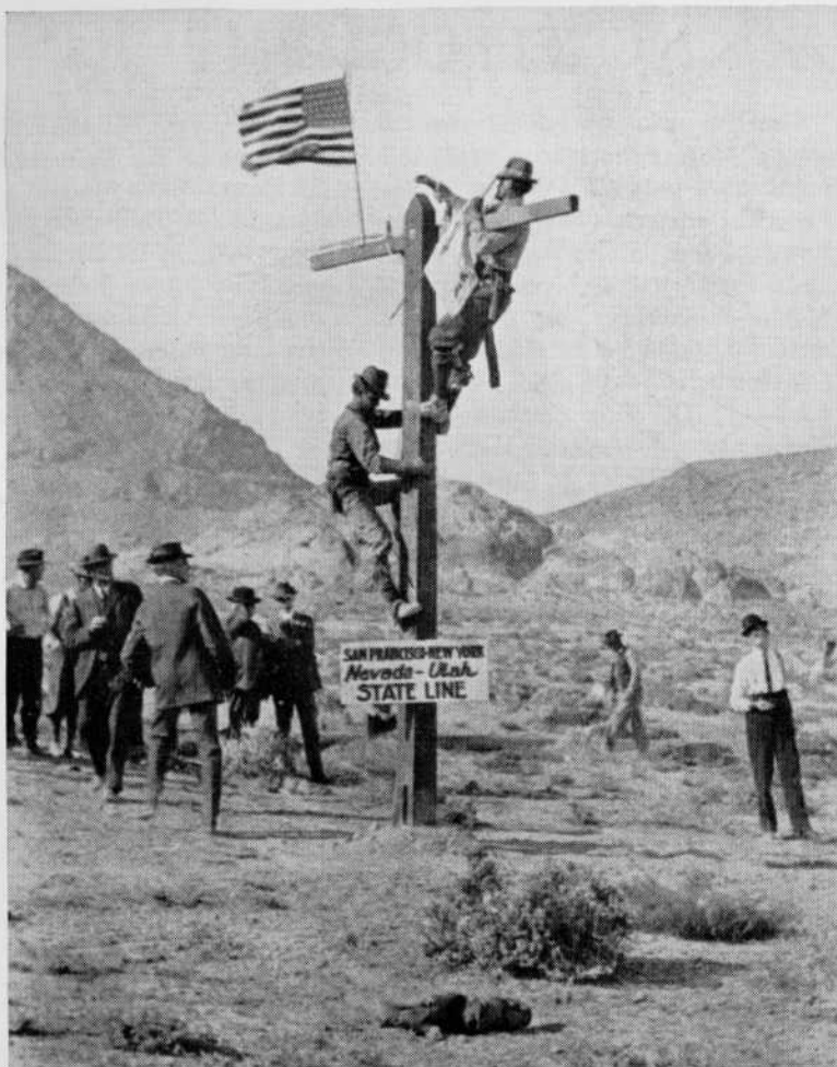
The first open wire line (linked here at the Nevada-Utah border) could carry only three calls and was vulnerable to interruptions.
