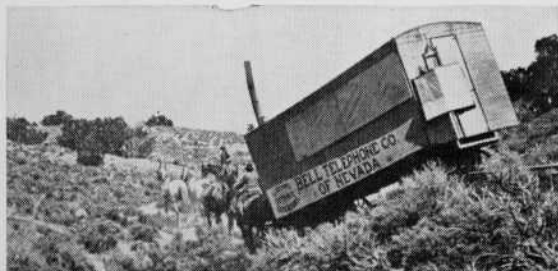
Installers of the first transcontinental line had to surmount hardships of windstorm, ice and scorching heat combined with rugged country.
